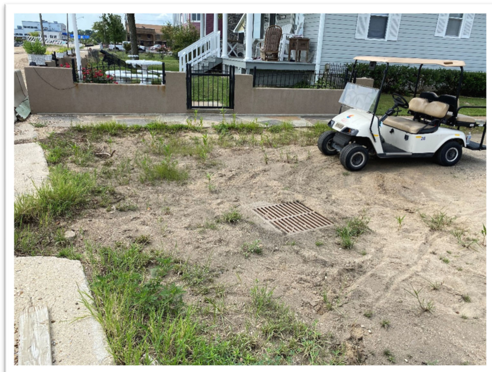
Photo 3: Stormwater inlet at end of Virginia Avenue, silted in from adjacent beach.
